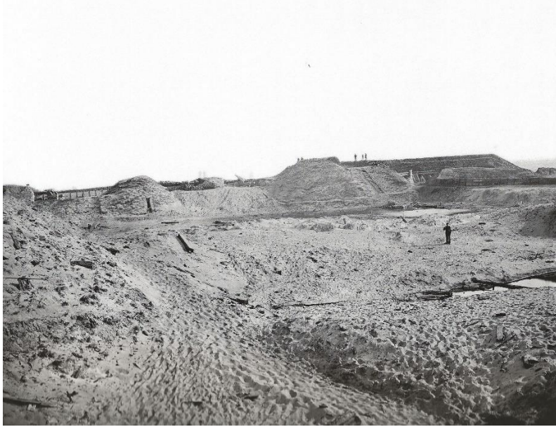
The Northeast Bastion from inside Fort Fisher. Center right, a soldier stands at the site of the main magazine that exploded the morning of January 16, killing about 200 people including Duncan McNeil. T.H. O'Sullivan, February 1865
